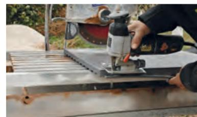
15. Cutting of the PUR using a jigsaw with laminate blade.
