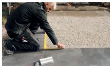
10. Check the angularity of the installed elements using a try square.
