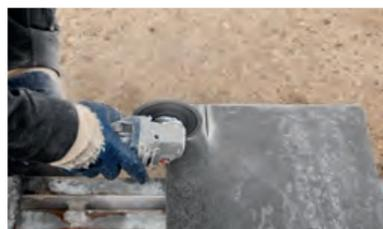
14. Any trimming of the elements is performed using a fine stoneware diamond cutting disc or wet cutter with extraction.
