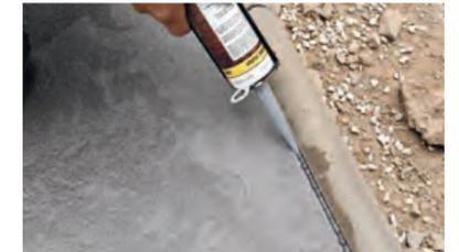
18. If required, the all-round edge expansion joints (at least 8 mm) can be filled with a suitable silicone. Ensure two-point adhesion in this case. Silicone joints generally require maintenance and must be checked and replaced at regular intervals.
