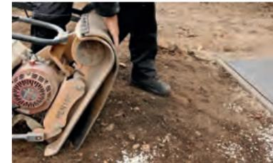
16. Compaction of the installed elements using a vibrating plate with a maximum weight of 60 kg and a 2-cm thick rubber pad.
