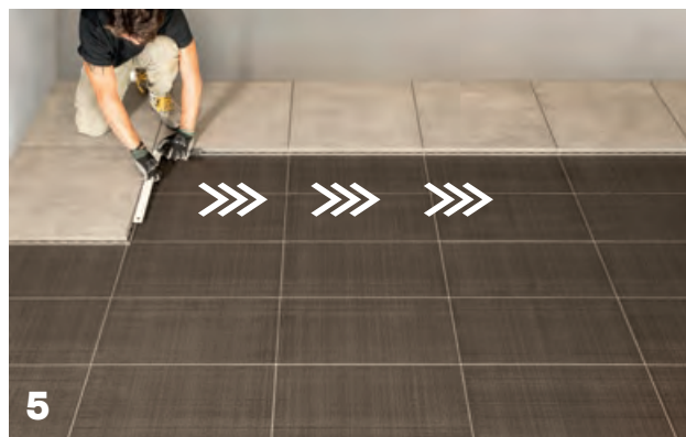
5 When the first row is complete, start again from the beginning, always ensuring that the elements are perpendicular.
