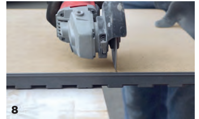
8 Elements can be cut with a tile cutter or angle-grinder.
