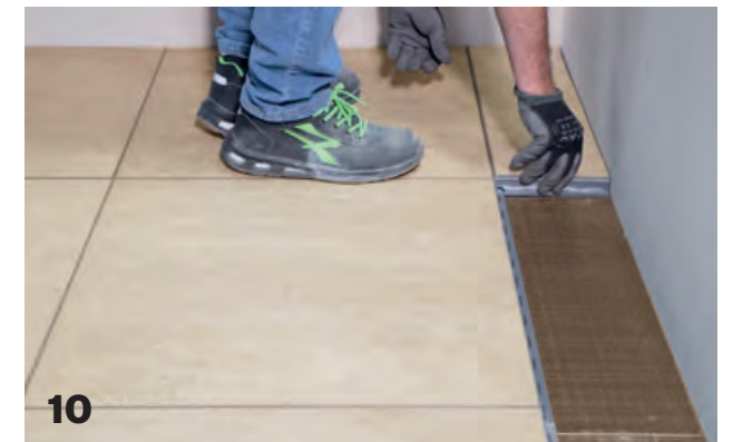
10 Fill any gaps between the elements and the wall with silicone.
