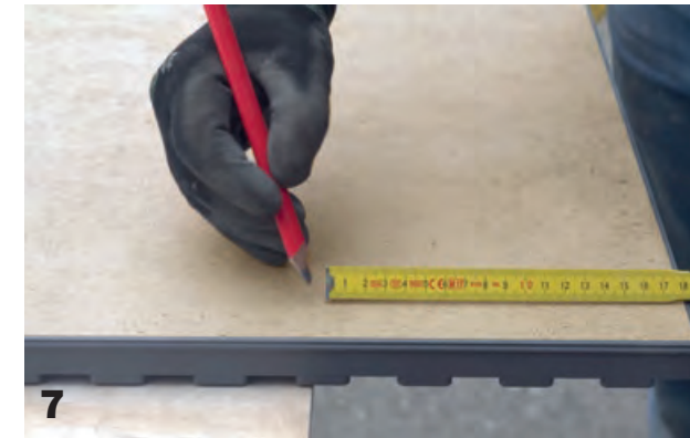
7 When done, cut elements to size around the edges if necessary.
